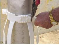
Regulations regarding the use of centralizers vary between states, however it is considered best practice to use one centralizer for each length of casing and screen. The Ground Water Well Licence / Bore Licence (if applicable) in many states also requires one centralizer for each length of casing.
