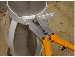
Note: The setting tool locks in behind the reinforced tabs at the rear of the female coupling. Open the jaws on the setting tool enough to reach the nearest tool lug and tension the centralizer collars enough to ensure that they will not move on the casing. Do not over tension the collars.
